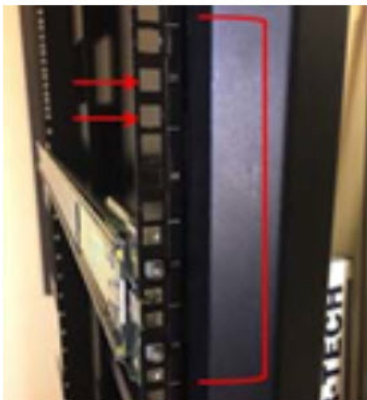
Rack post square hole location detail
